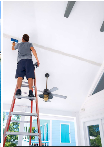
Marina Pavilion Paint
