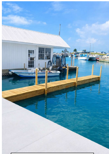
Marina Dock Repair
